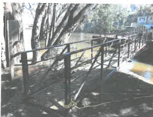
Photo Number 12 Gangplank to Timber Pontoon.
